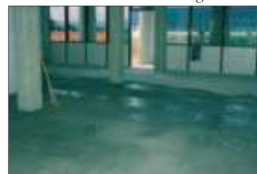
Floor foundation watering.
