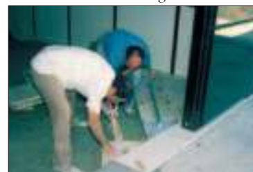
Mortar setting with high thickness.
