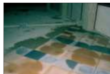
Daily watering at the end of the mortar setting.
