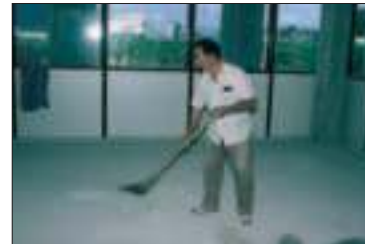
Floor foundation cleaning.
