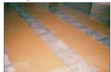
Joint's stuccoing (1 st colour).
